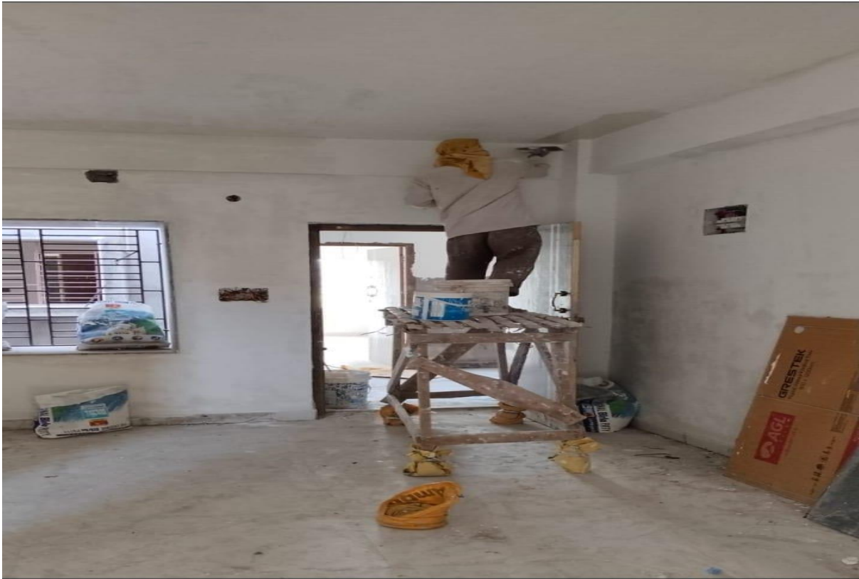
Putty work going on at 3C
