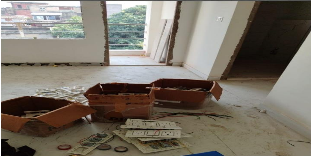
Switch board fitting going on at 3F
